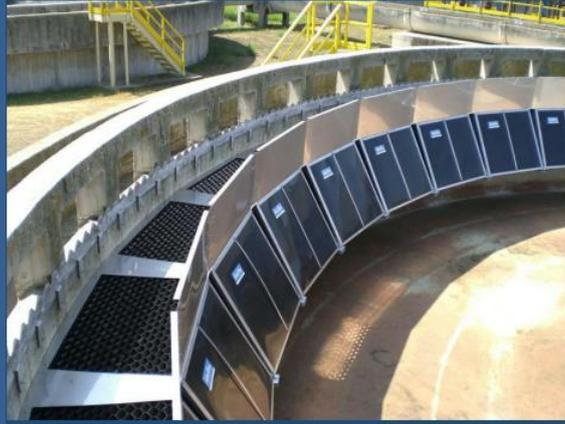
In circular tanks, installation of our lamella products is easy. It is the only solution for using them in circular geometric buildings because of their flexible structures.
