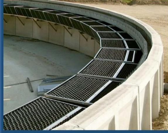
Particularly, in biological sinkage systems, in recent years, capacity increments and increase in efficiency have been provided by making lamella modul annexes with the aim to precipitate the mud with higher efficiency.
