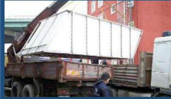
By making assembly of lamella moduls, they can be put easily into application area.
