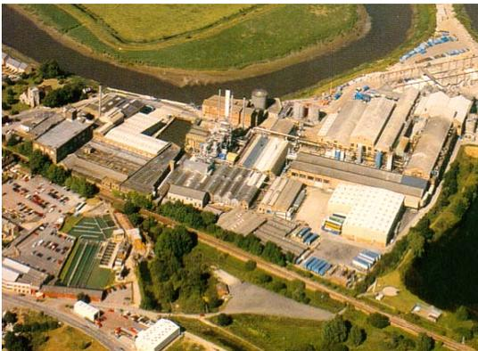
In 1994, Arjo Wiggins and Scottish HydroElectric together designed and constructed a gas turbine powered Combined Heat & Power Plant. The Plant is used to generate electricity and steam for the papermaking process. Surplus power is exported to the National Grid.
